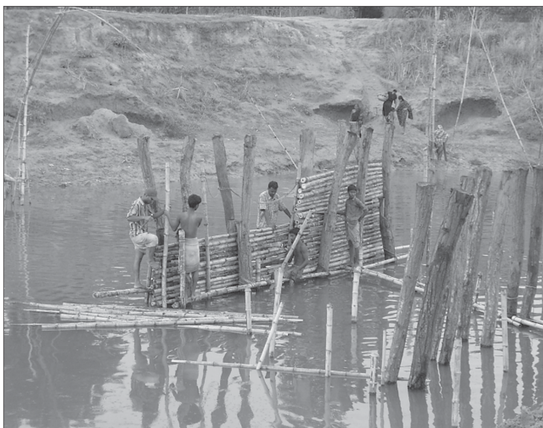
Fig. 6. Bottom vanes as low-cost river training structures for smaller rivers in Bangladesh
