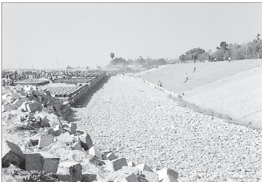
Fig. 5. Construction of FAP 21/22 bank protection along the Brahmaputra-Jamuna River in Bangladesh
